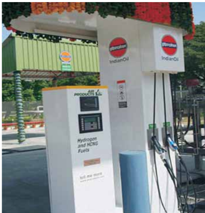
Fig.4: Hydrogen Dispensing Station set up at R&D Centre of IOCL at Faridabad
